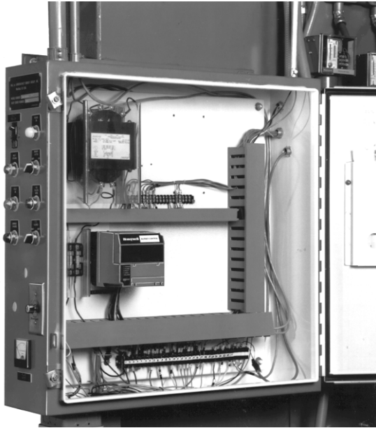
Fig. 11. Electrical panel installation.
